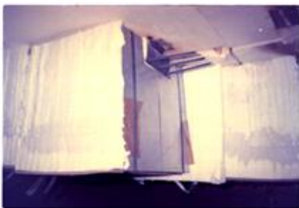
ALTRA® 72 Modules Roof Installation
